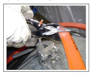
2. Notice the nylon cord in the pictures below. After cutting the belt make sure you have some gloves on when drilling out the nylon cord on both ends of the belt. (See photo below). Again using the VAR welding instructions and for non-reinforced VAR Belting skip to step 10 on the instruction sheet. If you have the <u>cord</u>, follow steps 3 through 9 of the instructions.
